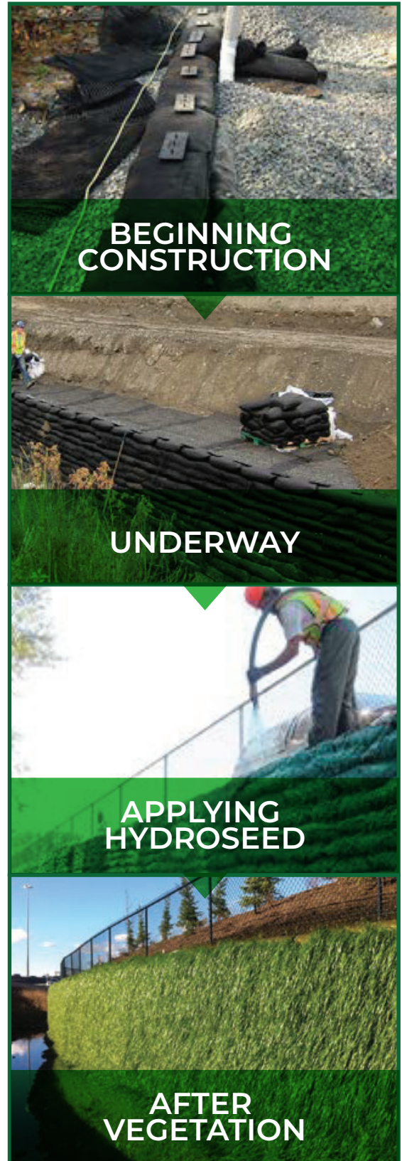
5m (16ft) tall commercial retaining wall
