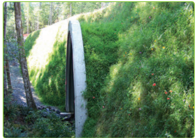
10m (33ft) tall municipal roadway
